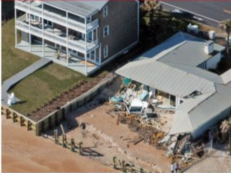
Two properties side-by-side that show how stronger building codes can protect properties
