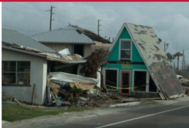
Damage caused by Hurricane Michael in Mexico Beach, FL Source: Shutterstock
