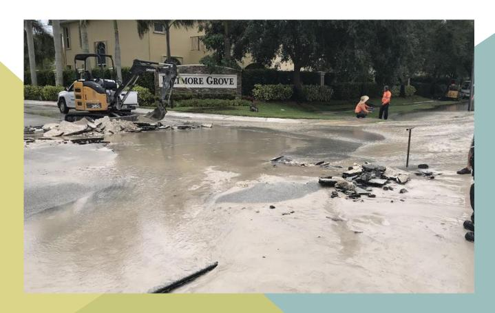
May 12, 2018, contractor for a wireless carrier installing fiber via directional bore struck a water main, which caused a flood and the road collapsed, creating a sink hole which blocked the entrance to a neighborhood in Cooper City. (Sun Sentinel picture)
