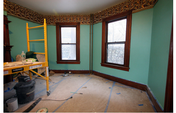
Restoring a historic house (via Flickr )
